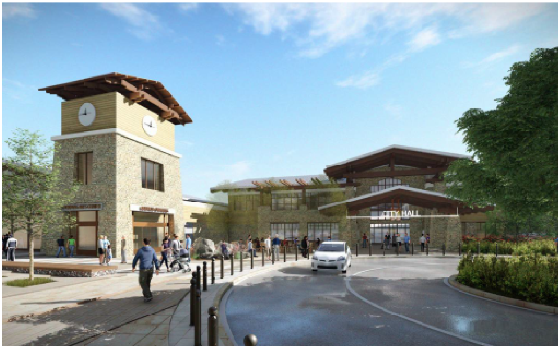
Figure 5 View of Future Lake Forest Council Chamber/Performing Arts Building and City Hall
