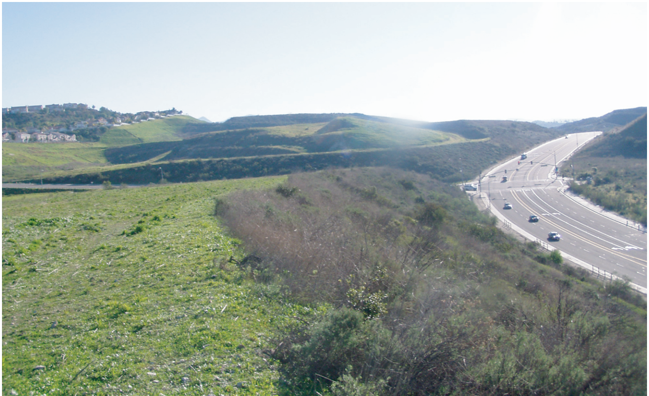
Graded East and West of Saddleback Ranch Road, North of Glen Ranch Road
