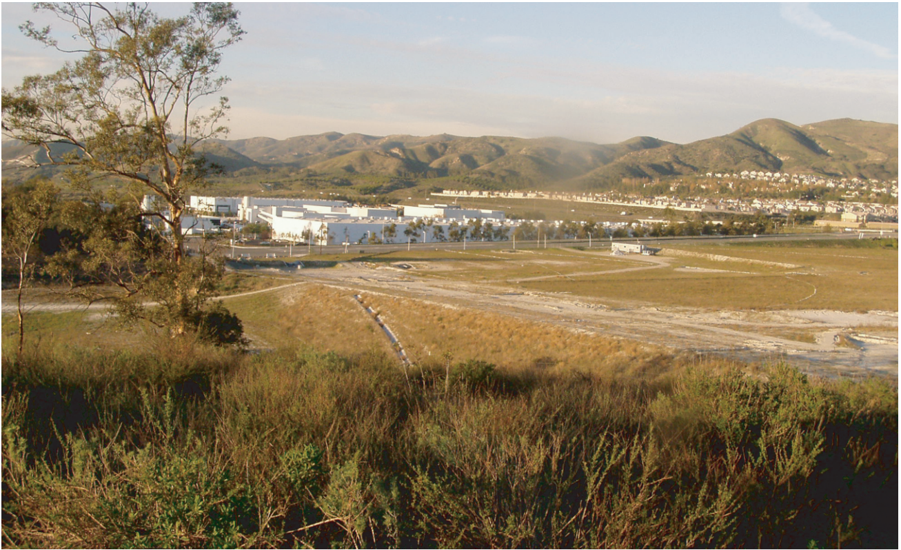
Graded Area in Northern Portion
