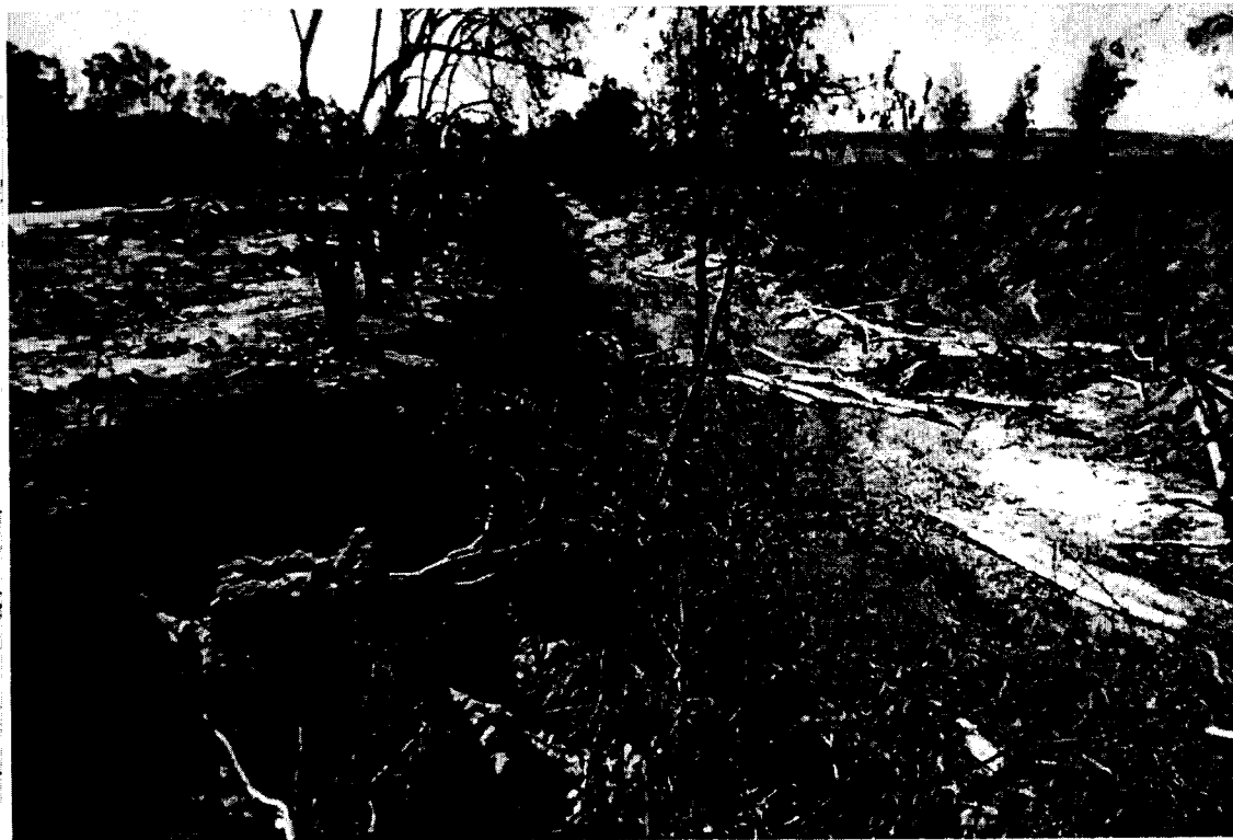
Figure 7. Incised channel upstream from drop structure, December, 1998. A. Looking upstream near Profile 4AA. Note failed bank on far side. B. Looking downstream near Profile X.
