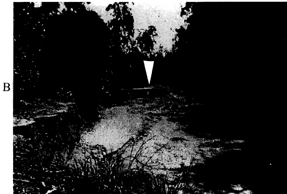
Figure 6. Looking downstream just below Profile 3. A. 1991. Note channel is still roughly trapezoidal. B. 1992. Channel has eroded the left bank by several meters removing the road and the first row of orange trees. The bank is 6 feet (2m) high. Note person standing by bank (arrow.)
